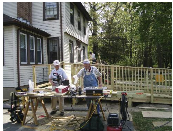
SPAN ramp construction in progress.
